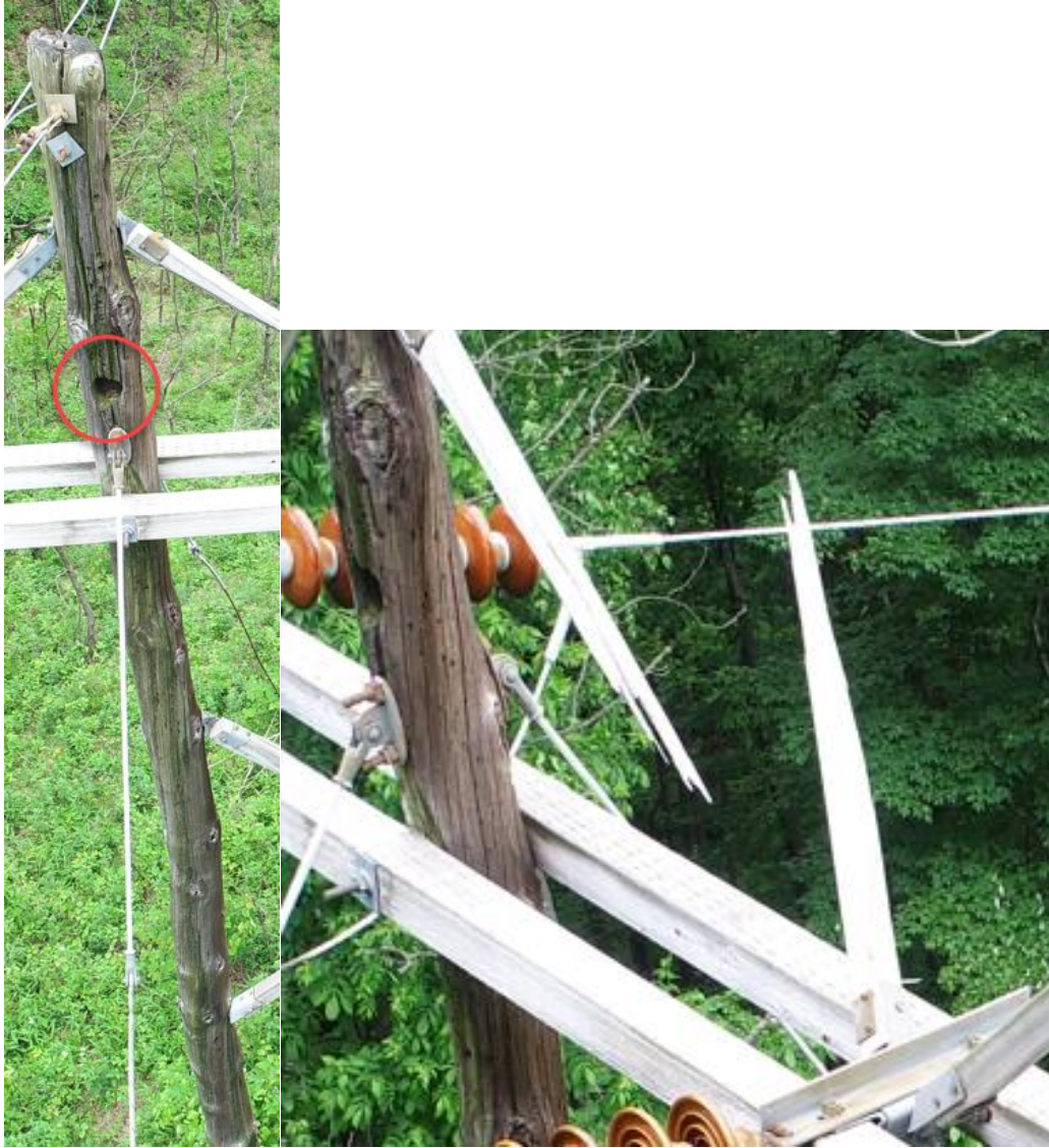
Figures 11 and 12: Component 2: Floyd – Stuart 69-kV Line Structure 452-45: Large Pole Cavity, Pole Decay, and Broken Knee Brace
