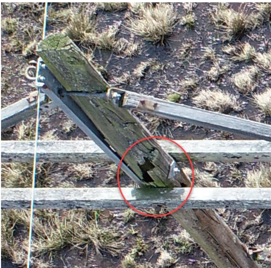
Figure 18: Component 3: Claytor – Fieldale 138-kV Line Structure 30-114: Severe Upper Pole Splitting Impacting Structural Integrity at Crossarm Attachment Point
