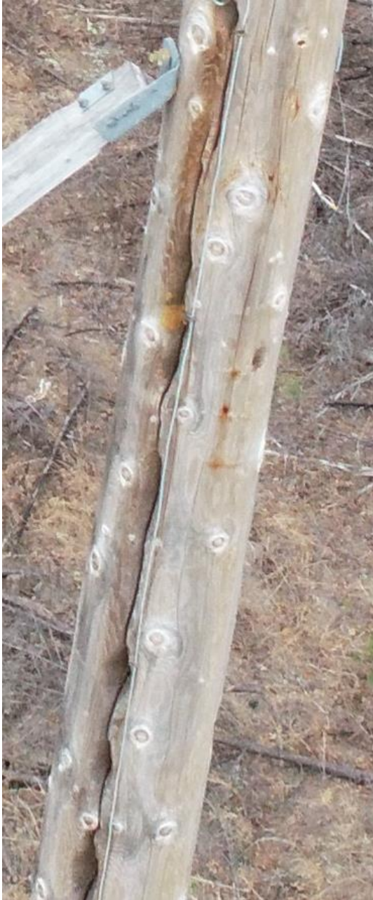
Figures 23 and 24: Component 3: Claytor – Fieldale 138-kV Line Structure 30-218: Moderate Vertical Pole Splitting and Flashover/Arcing Damage to Insulator
