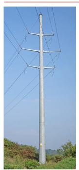
Crews plan to build less than a quarter of a mile of transmission line, on Appalachian Power property, to connect the new substations to existing lines. Plans call for using single steel poles when building the line.
