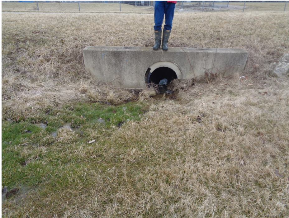
Photograph 9. View of culvert associated with upland drainage feature just south of Project area. Photograph taken facing east.
