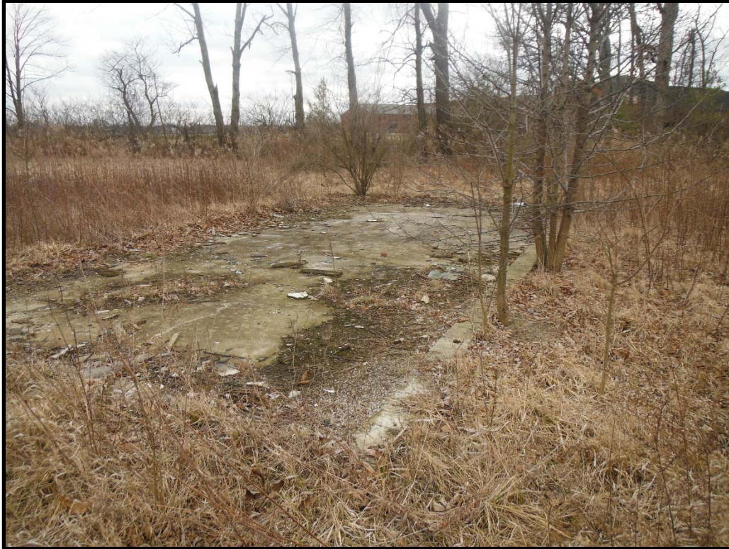
Figure 12. View of existing foundation.
