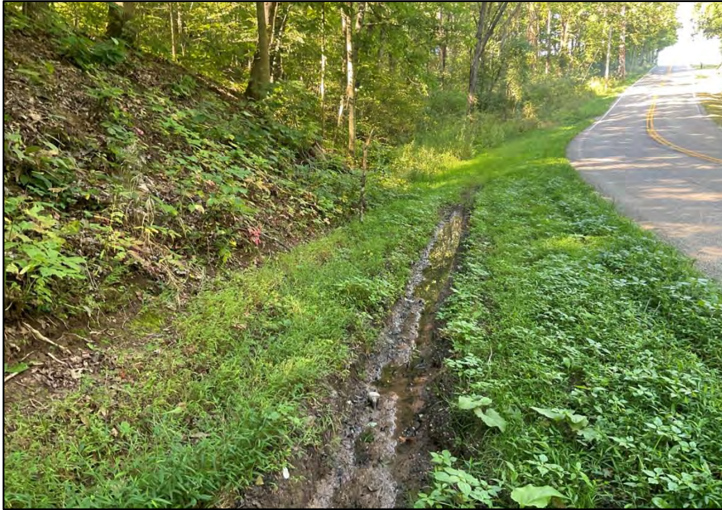
Photograph 329. Stormwater Erosion SWE-AGS-012, Facing Southwest
