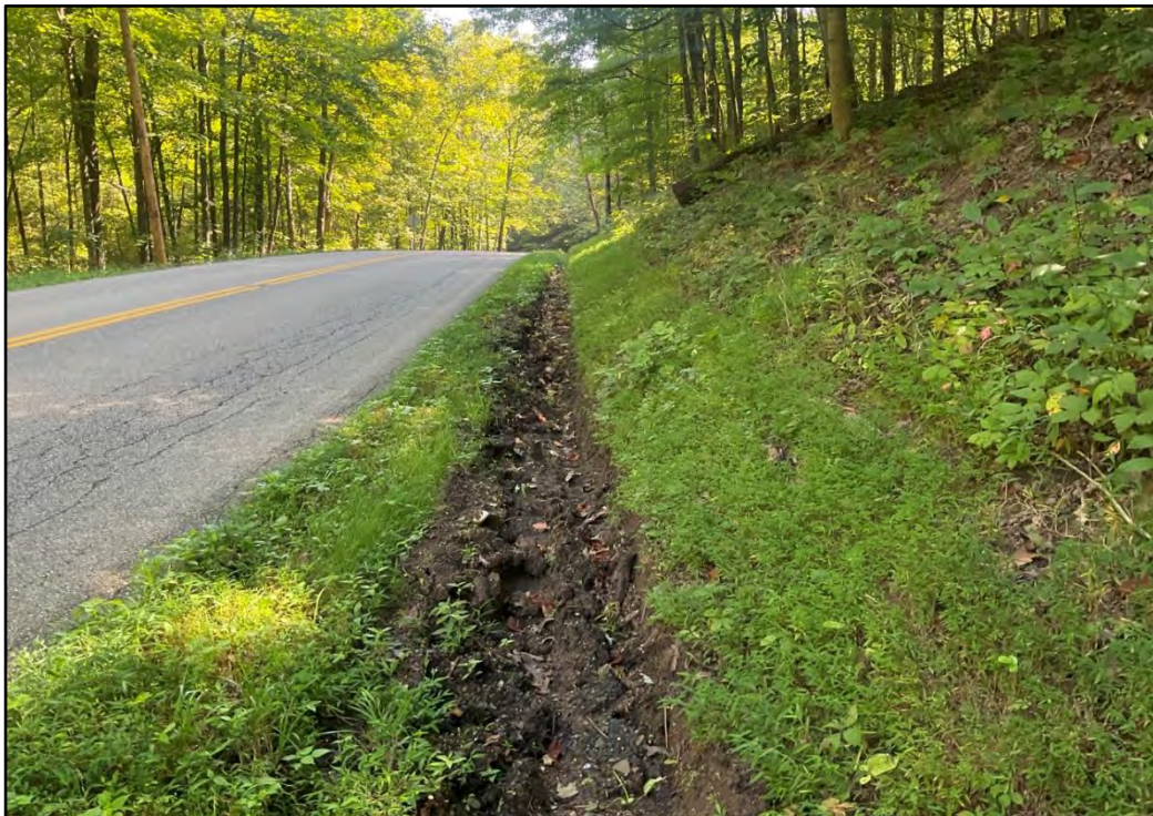
Photograph 330. Stormwater Erosion SWE-AGS-012, Facing Northeast
