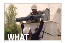
Improvements involve upgrading approximately 20-miles of 138-kilovolt transmission line by replacing lattice towers with steel monopoles and new wire.
