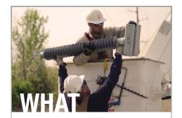
I&M is rebuilding approximately 10-miles of 69-kilovolt (kV) transmission line. Existing wood poles will be replaced with steel monopoles and new wires of the same voltage.
