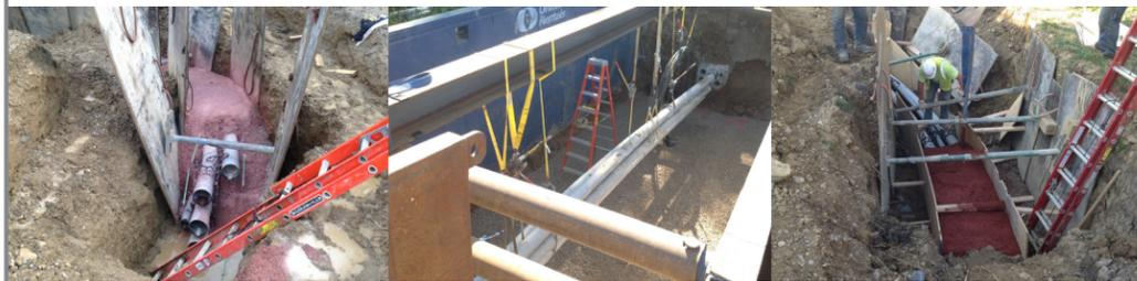
**3 Vault installation and cable pulling:** Crews may install vaults – large concrete boxes with manhole covers – at regular intervals along the route. Afterward, cable is pulled through the conduit system and spliced together.
