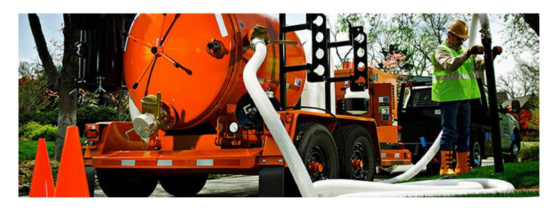
Hydro Excavation: Crews use hydro excavation (hydrovac) in areas where many underground utilities are located near each other. This process involves using pressurized water to break down soil to expose underground utilities. Afterward, crews backfill the area. The process helps prevent damage to underground infrastructure while gathering important information.
