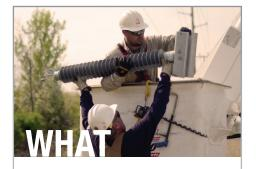
The existing 69-kV transmission line will be replaced and upgraded with 138-kV lines and structures. These 138-kV facilities are slightly taller and heavier and will allow the lines to carry more current and help meet customers' increased demand for power. The company will relocate and expand the existing Barnesville Substation.
