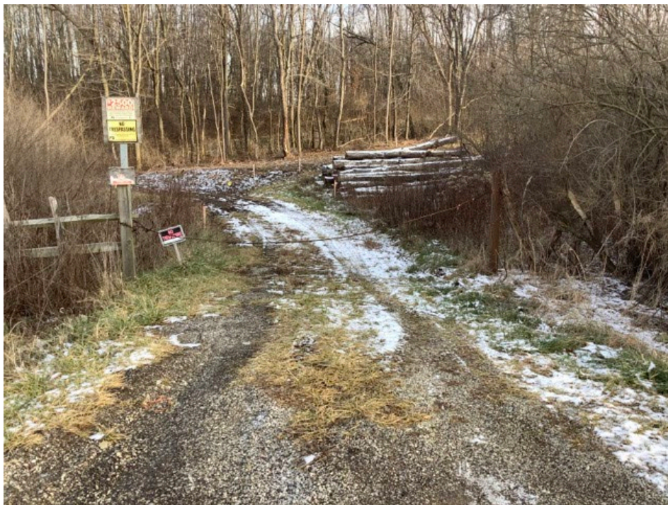
Photograph Location 4. Representative view of existing gravel road within the Project area. Photograph taken facing east.
