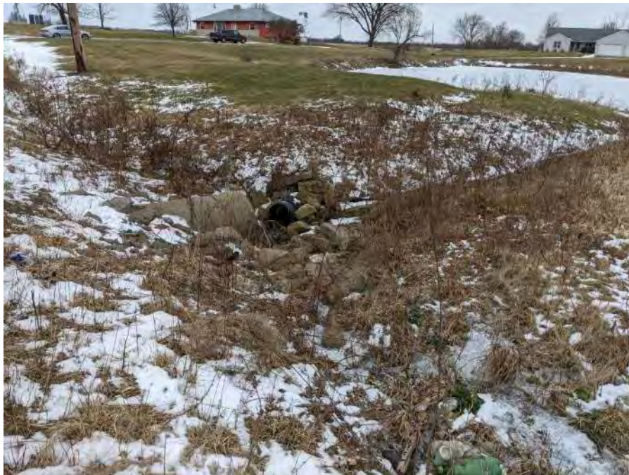
Photo 2 - Area A Pond 5 – Looking south along Mink St. roadway ditch (EMH&T, 1/21/2022)
