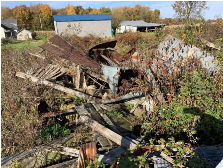
Photo 10 - Area E Overgrown/Avoided area behind farmstead – debris pile (EMH&T, 11/4/2021)
