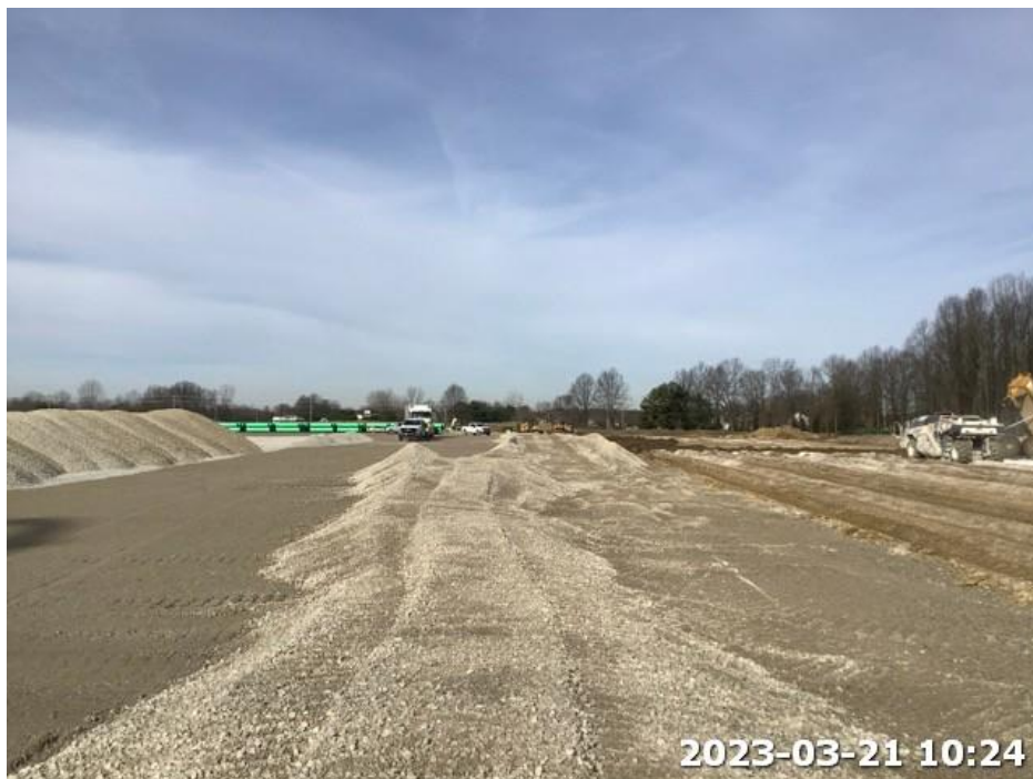
Photo 6. View of grading activities in southeast corner of Project area. Photograph taken facing west.
