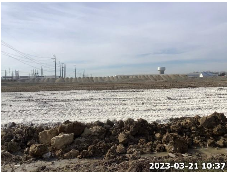
Photo 4. View of grading activities from northern edge of the Project area. Photograph taken facing south.
