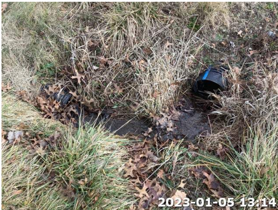
Photograph Location 5. Representative view of existing culvert within the Project area. Photograph taken facing east.
