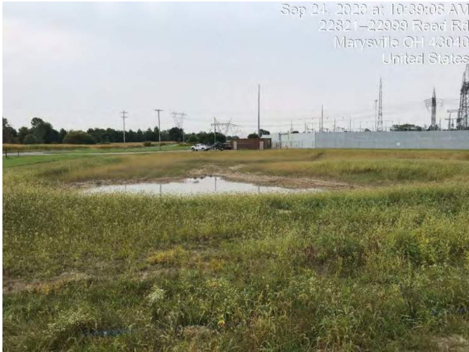
Photo Location 11. Representative view of recently constructed stormwater detention basin and new field habitat area. Photograph taken facing south.
