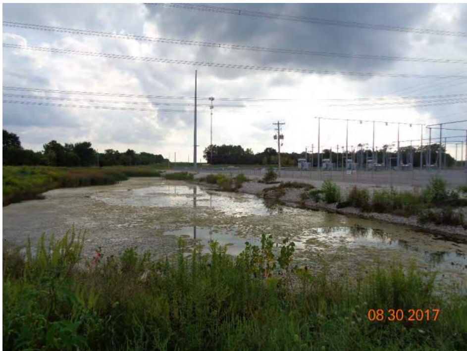
Photo Location 11. View of Wetland 8. Photograph taken facing southwest.
