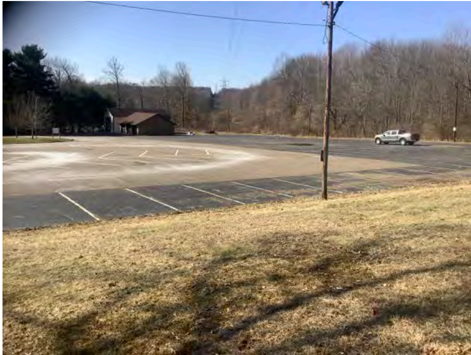
Photograph Location 6. Representative view of existing paved roadway/surface. Photograph taken facing southwest.
