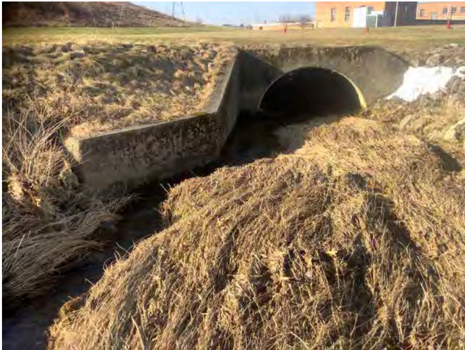
Photograph Location 43. View of downstream portion of Stream 5. Photograph taken facing downstream/southwest.
