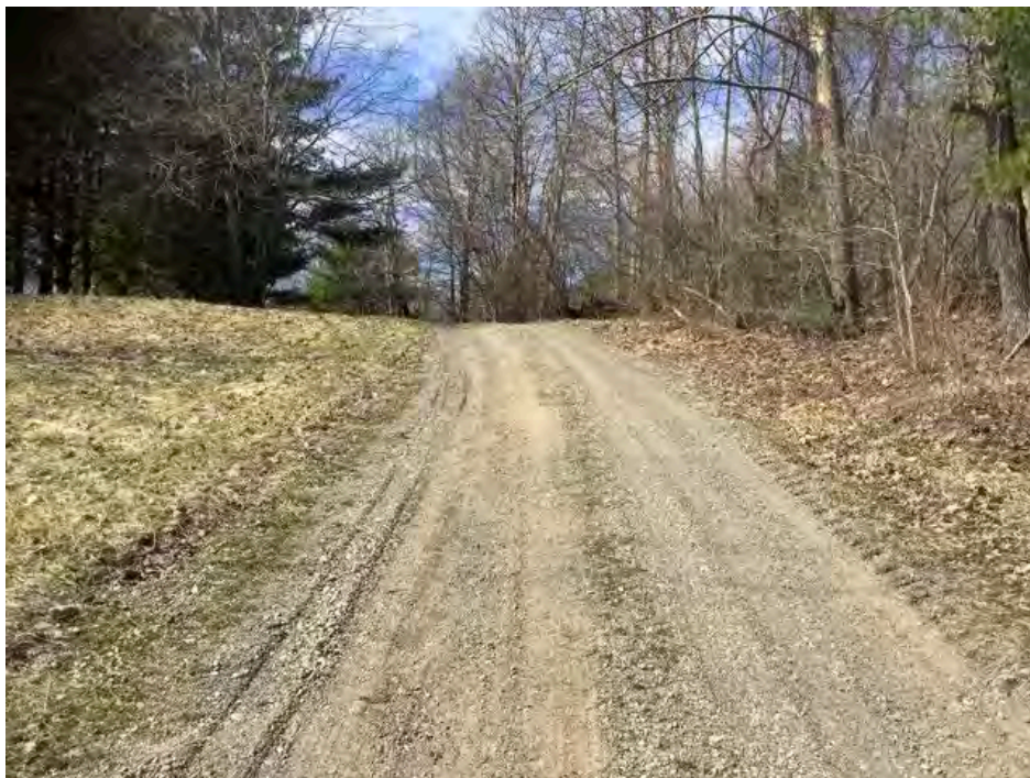
Photograph Location 4. Representative view of existing gravel drive. Photograph taken facing west.
