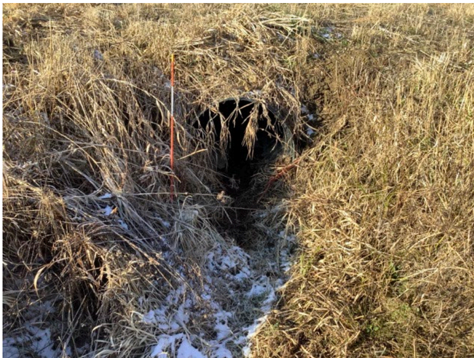
Photograph Location 2. View of Stream 18 and existing culvert. Photograph taken facing downstream/west.
