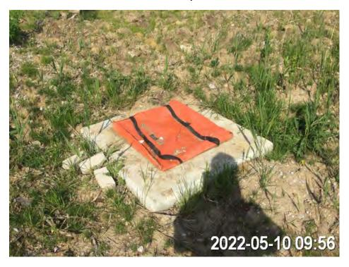
Photo Location 11. View of storm drain with inlet protection. Photograph taken facing west.
